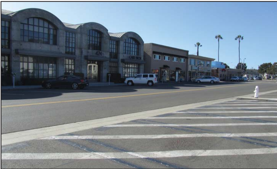
View of mixed commercial uses to the south of the project site.
